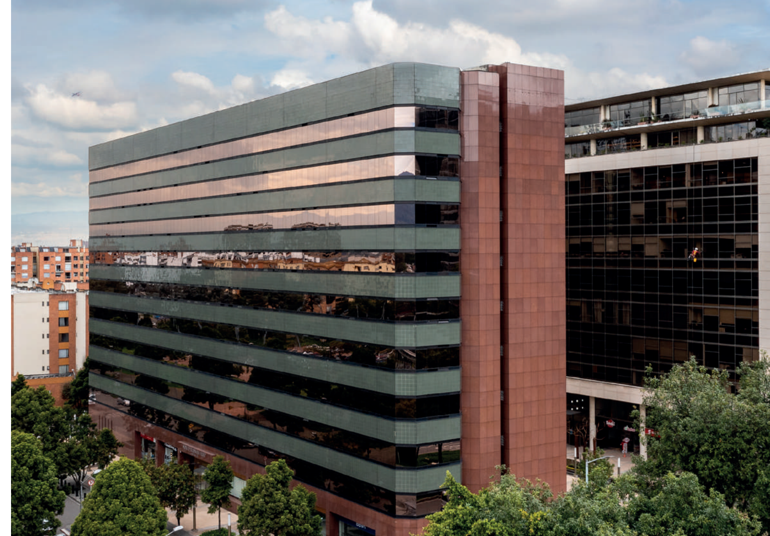
EDIFICIO WORLD BUSINESS PORT -Bogotá
